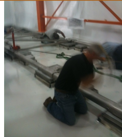
Using a come-along tool and a little elbow grease to square the frame
